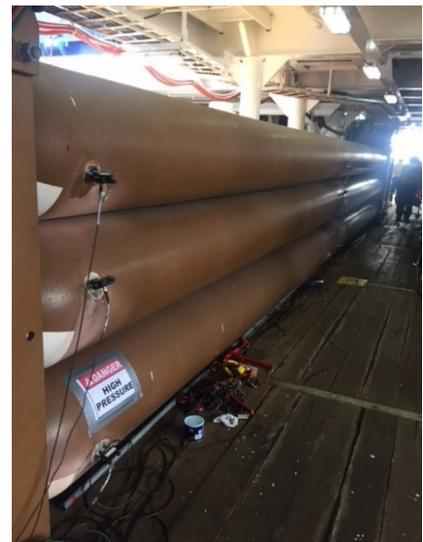
**Fig 1: Sensors mounting at Kelly tubes**
