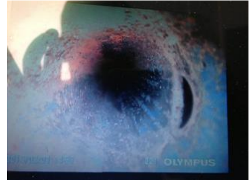
Video scope Images of Defective Tubes
